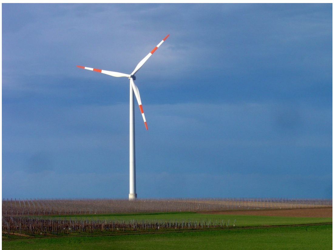
Figure 4: Large scale wind turbine
