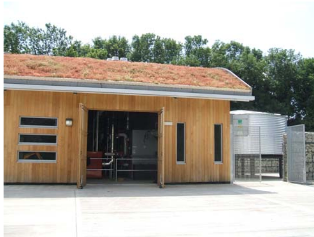
Betteshanger Colliery, Kent 1 MW district heating
