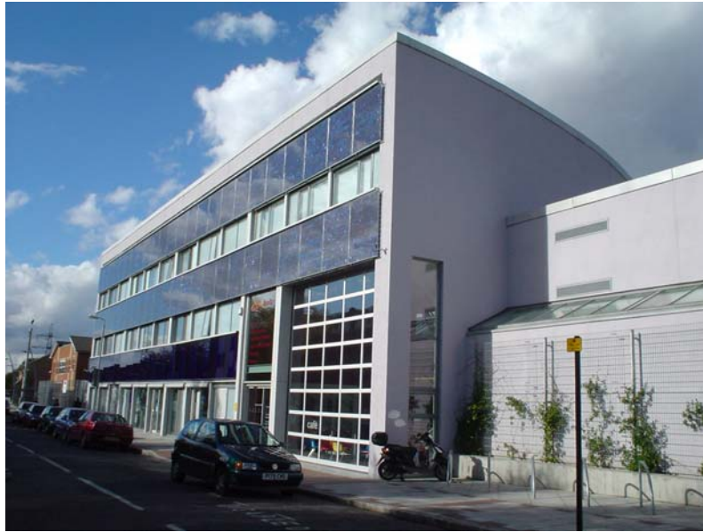
Figure 13 - Photovoltaic Systems on The Hub, Newham, London
