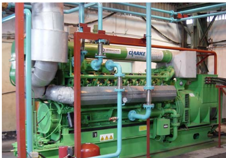
Figure 9 - A typical natural gas CHP engine
